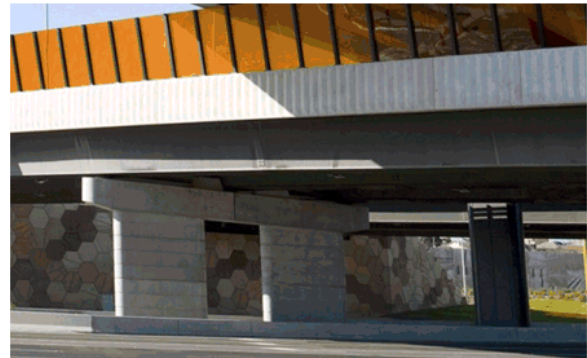
East Link - Use of rounded edges to the headstock and narrowed blade piers softens the form of the overall structure.
