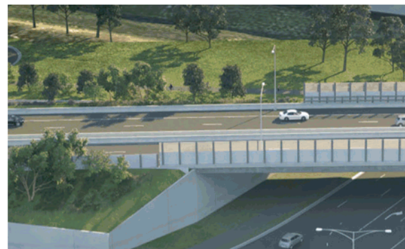
The proposed interface between noisewalls above shows an abrupt transition. (source: https://roadprojects.vic.gov.au/projects/mordialloc-freeway/view-the-ees ). Transitions should taper and integrate with adjacent forms (refer image 2 Deer Park Bypass) or continue at a consistent height rather than creating a sudden drop as pictured above.
