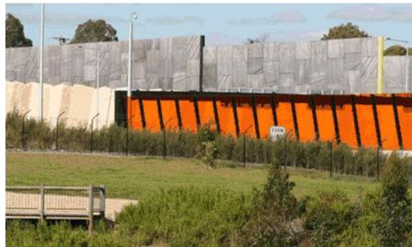
East Link - Transparent noise walls to be used adjacent to open space.
