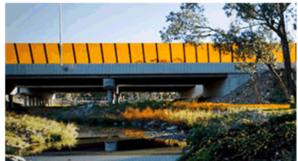
East Link - Plexi-glass panel noise walls are consistent in height rather than stepped.
