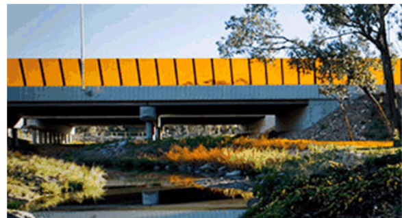
East Link - Plexi-glass panel noise walls are consistent in height rather than stepped.
