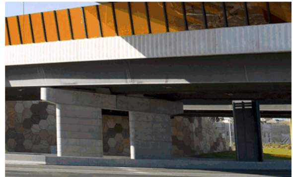
East Link - Use of rounded edges to the headstock and narrowed blade piers softens the form of the overall structure.
