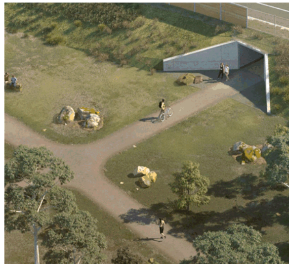
Proposed pedestrian underpass at Braeside Park - Aerial view (source: https://roadprojects.vic.gov.au/projects/mordialloc-freeway/view-the-ees ). Narrow entries create a dark, inhospitable and potentially unsafe environment.
