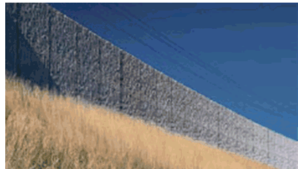
3. East Link - Walls should be a consistent height wherever possible, as pictured above.
