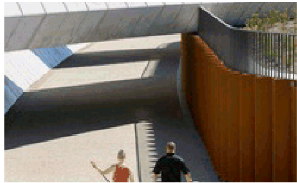
Bowen Place - Canberra. Natural light to central underpass
