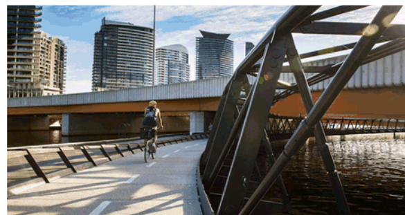
Jim Stynes Bridge. Clear view lines through underpass.
