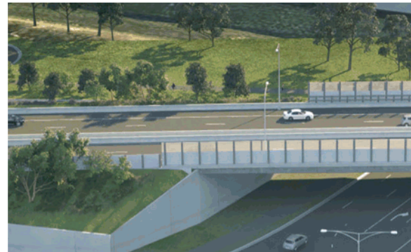
The proposed interface between noisewalls above shows an abrupt transition. (source: https://roadprojects.vic.gov.au/projects/mordialloc-freeway/view-the-ees ). Transitions should taper and integrate with adjacent forms (refer image 2 Deer Park Bypass) or continue at a consistent height rather than creating a sudden drop as pictured above.
